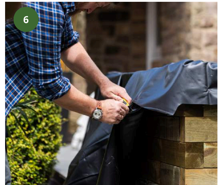
Trim away some excess - to make adjustments easier, carefully trim away some overhanging liner (leave plenty).
